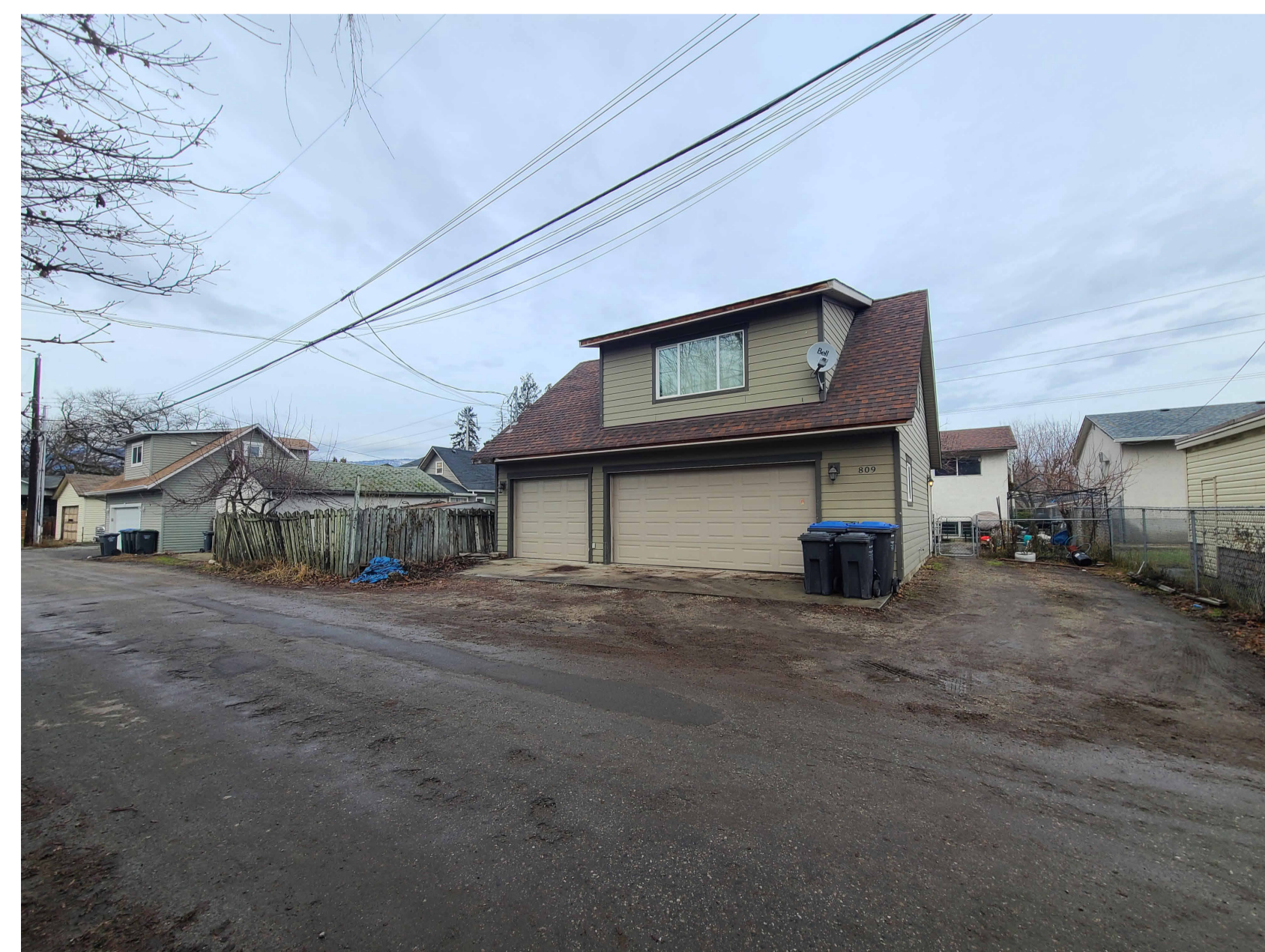
4. VIEW FROM THE LANE FACING THE SITE, TOWARDS RICHTER STREET
